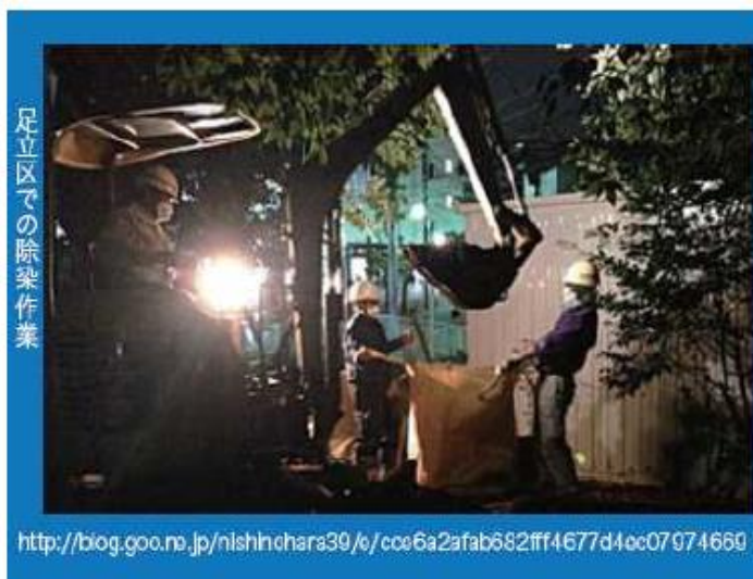
Photo: Nighttime decontamination work in Adachi ward, Tokyo
